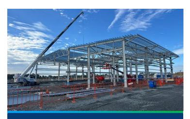
**Image:** More than 150 tonnes of structural steel framework has been erected for the main building (August 2025).
